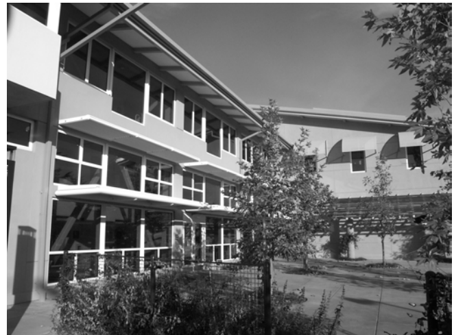
Fig. 3: The south shading overhangs and light shelves. In the distance shading of the west-facing faculty offices. (Photograph by D. W. Aitken.)
